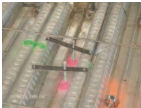
Figure 25: Visual control with color coding to show locations for sheet metal straps and pipe hangers in metal decking (Figure 2 in Tommelein 2008, source: John Mack, Southland Industries, Inc., presentation at 2007 Annual Conference of the Lean Construction Institute, San Francisco, CA)
