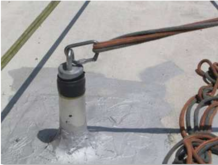
Roof anchors
