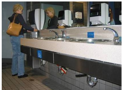
Figure 15: Sink with Adjustable Apron at Oakland Airport, California (© 2004 Iris D. Tommelein)
