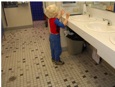
Figure 14: Sink with Cut-out Apron in San Francisco Airport, California (© 2007 Iris D. Tommelein)
