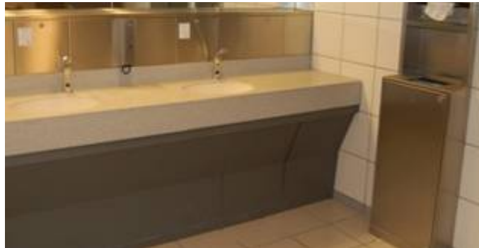
Figure 13: Sink with Covered Apron in Brussels Zaventem Airport, Belgium (© 2007 Iris D. Tommelein)
