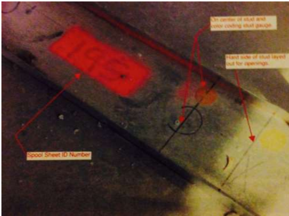
Figure 97: Spool Sheet Framing Layout
