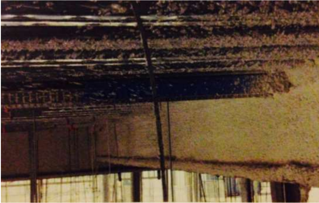
Figure 92: Masking Top Track Prior to SFRM
