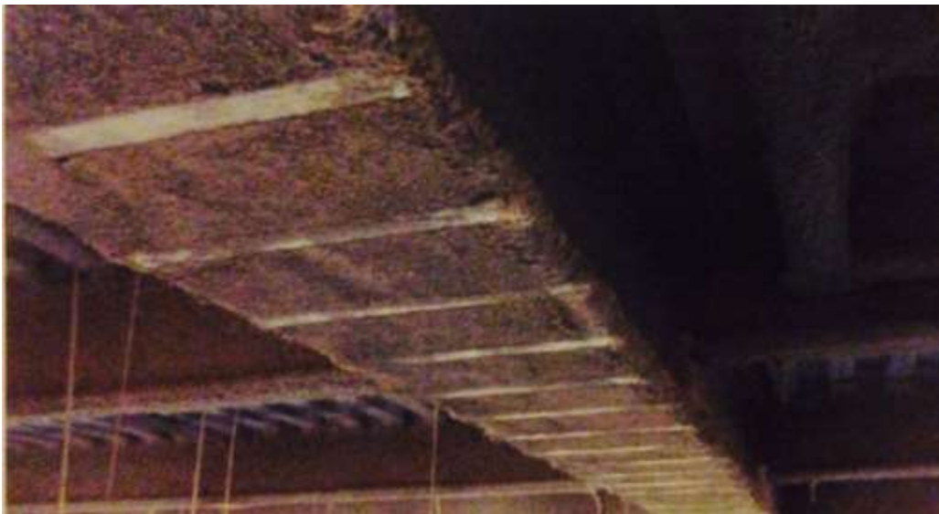
Figure 93: Screeding Z-Clips
